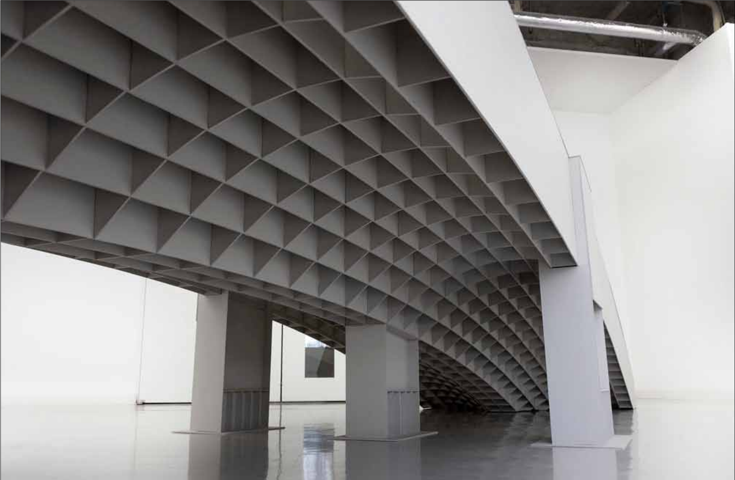
Przemysław Jasielski – Paper Bridge Over Stone River Materials: paper, Dimensions: 550/130/60 cm, 2012, Fully functional bridge made entirely out of paper. The design was created basing on the traditional Japanese bridges built at the entrance to the temple grounds. Viewers were invited to have a walk and test the strength of the construction.
